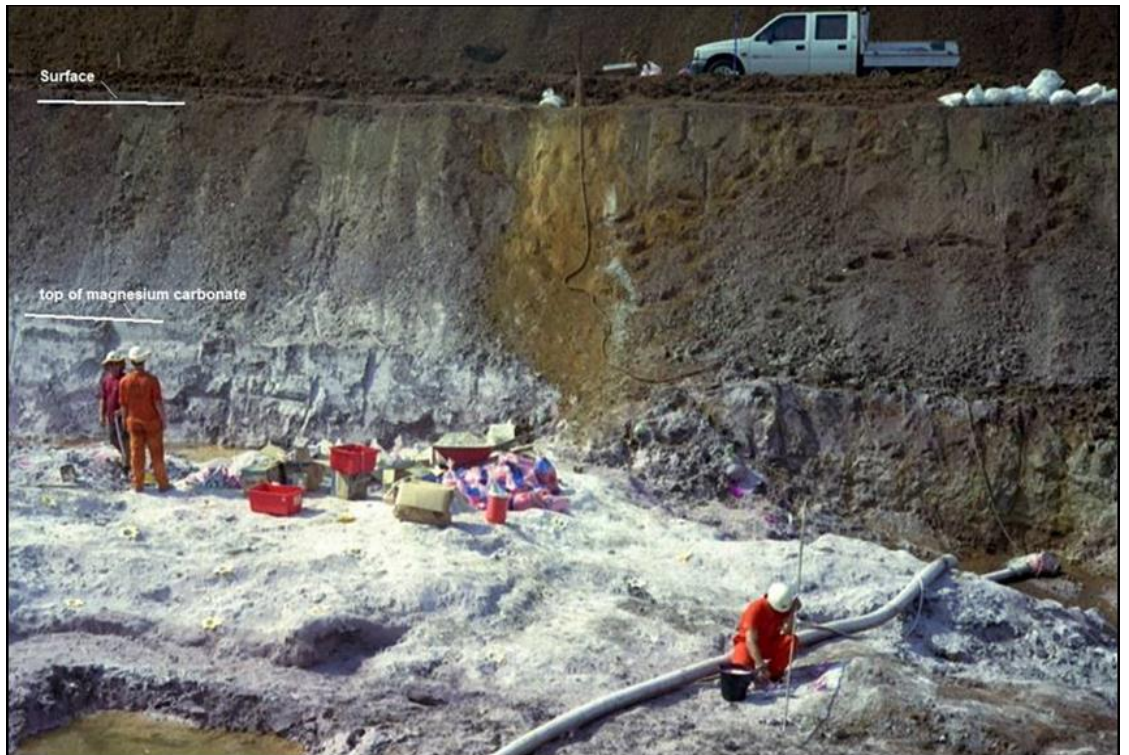
Figure 13 Test mining of magnesium at Winchester during the wet season (preparing to blast Level -1)
